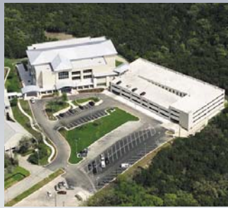
Training and Technology Building & Parking Garage Region XIII Education Service Center 168,000 Sq. Ft.
