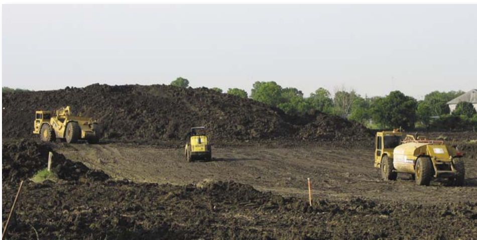
In order to complete a parking lot similar to the above photo, extensive excavation, hauling and compaction is required (see photo below).
