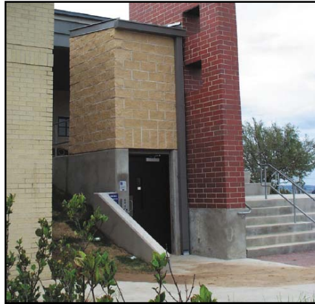
A wheelchair lift was more economical than extensive ramps.
