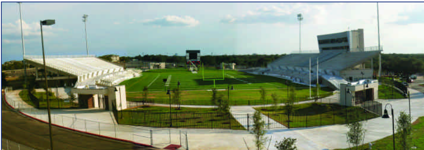
The new Round Rock ISD Stadium Complex, will service four area high schools and has room enough for 11,000 spectators.
