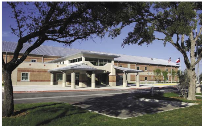
Rutledge Elementary has won three awards - ABC's Excellence in Construction, Texas Construction Magazine's Award of Excellence and TCA's 2006 Achievement Award.
