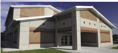
Several different concrete textures and colors were used to vary the design.
