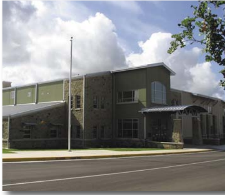
Several different concrete textures and colors were used to vary the design.
