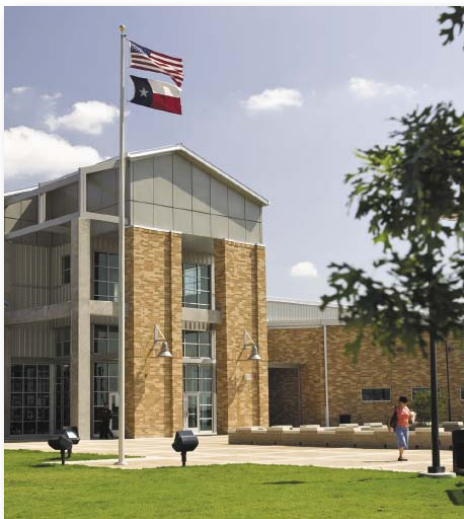
Several different concrete textures and colors were used to vary the exterior design of the new San Marcos High School.
