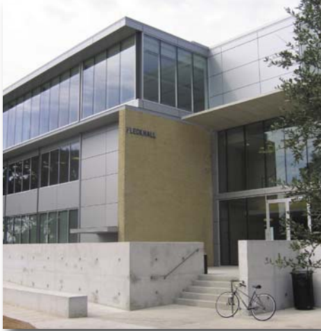
By working with city officials, St. Edward's University Fleck Hall Renovations and Additions' first two floors opened for the beginning of the school year and the third floor conference rooms one month later as planned.
